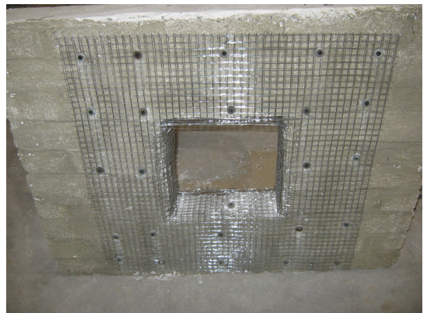
Figure (7) Details of the used rehabilitation technique using (2, 3, 4) layers of steel wire mesh fixed with fisher bolts.
