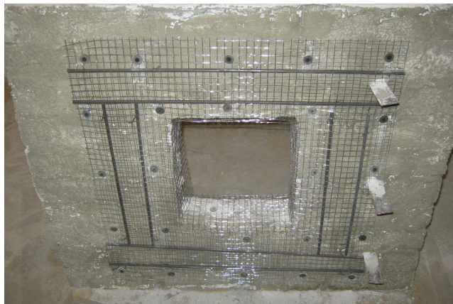
Figure (10) Details of the used rehabilitation technique using two layers of steel wire mesh with 206 additional external steel bars in between.
