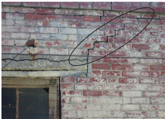
Figures (1) and (2) The cracking through the masonry developed primarily along the mortar joints in a diagonal stepping pattern
