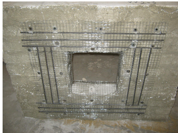
Figure (11) Details of the used rehabilitation technique using two layers of steel wire mesh with 306 additional external steel bars in between.
